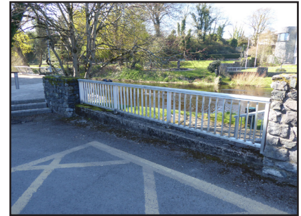
Image 003: Community built walls and railings on Market Square
