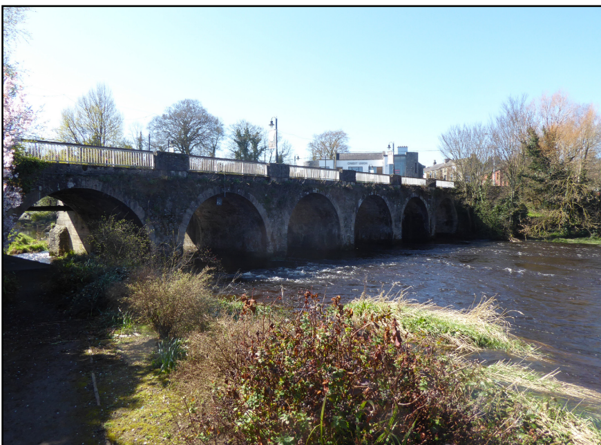
Image 001: Kilcullen Bridge from the North
