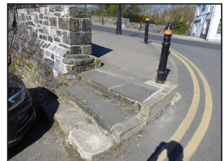
Image 011: Existing surfacing at Market Square
